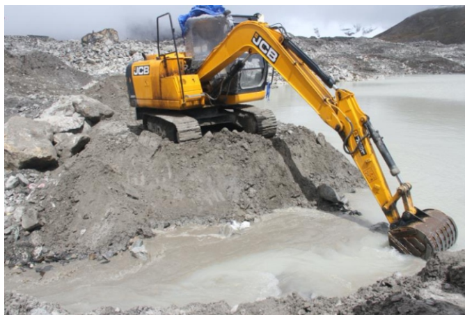
Figure 4.4: Artificial Channel Enlargement of Imja Lake, Nepal, 26 September 2016 (Source: UNDP). (Artificial channel enlargement for lake level lowering is a very critical moment, as it can lead to the formation of a breach and a GLOF/LLOF)
