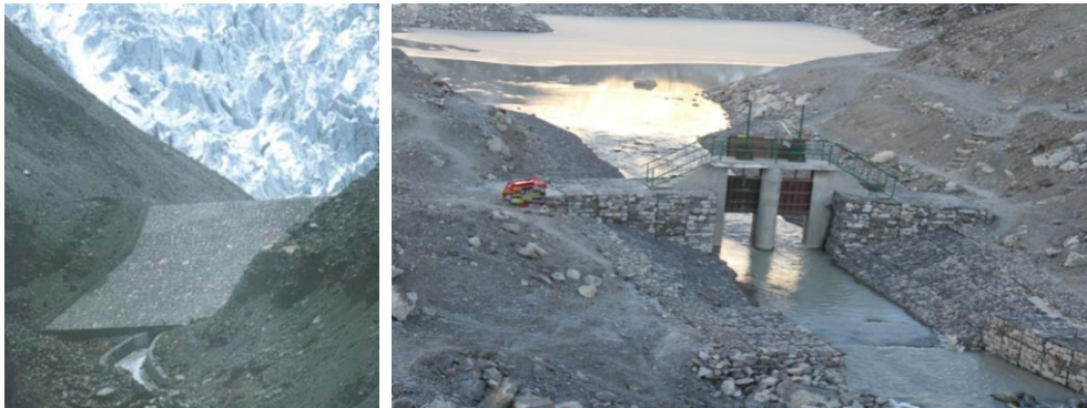
Figure 4.5 : (a) Outlet channel with reinforced dam reconstruction at the moraine dammed lake Laguna Cuchillacocha, Peru (Photo: C. Portocarrero), (b) Open channel at Imja Lake, Nepal, inaugurated in October 2016 (Photo: UNDP).
